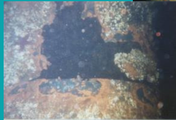
Corrosion of Underwater Structures captured by Camera
